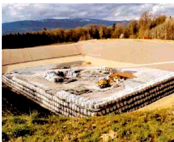
Fig. 5.2 The Swiss residual material landfill Oulens VS. The blocks of solidified incinerator filter ashes are visible
